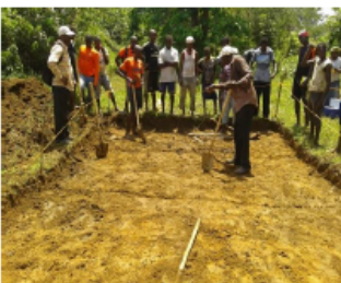
Clearing Topsoil
