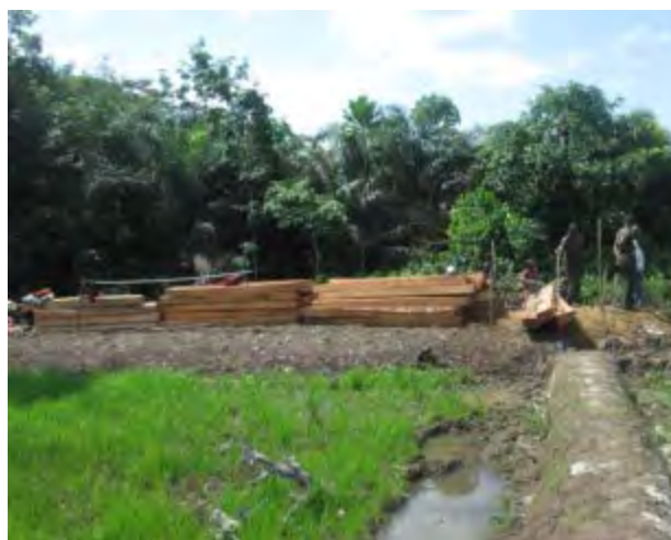
Figure 2: Spillway construction at Marmeï Farm, Nimba County.
