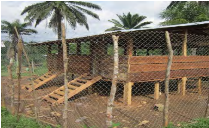
Figure 6: Completed goat shelter at Zodoie Farmers Association site in Nimba County.
