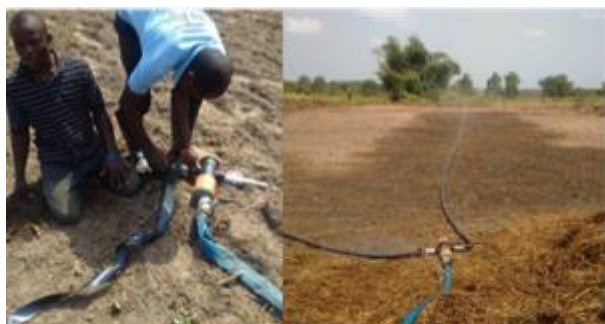
Figure 3: Installing and testing a sprinkler irrigation system, Mount Barclay, Montserrado
