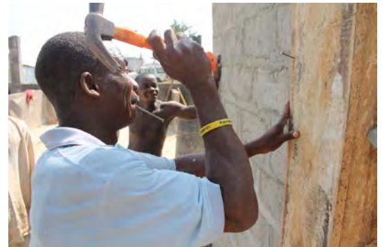
Construction worker sets support boards at the CARI quarantine facility.
