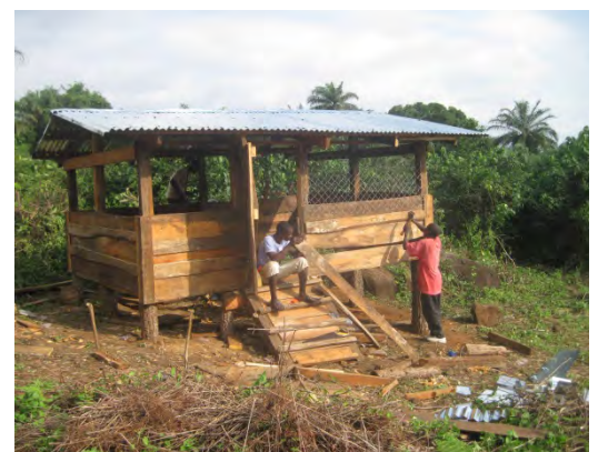
Goat shelter construction in Buchanan, Grand Bassa County.
