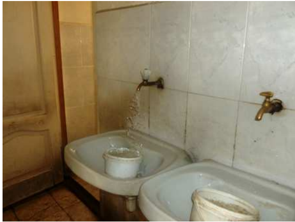
Poor sanitary conditions in the factory's WCs.
