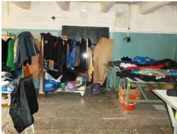
Blocked emergency exit.
