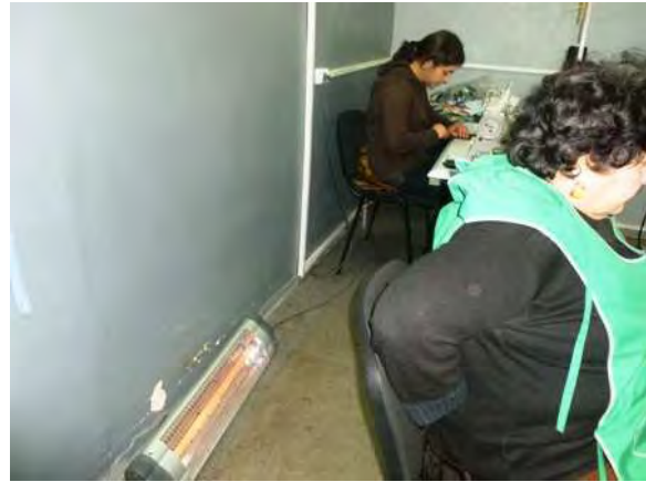
Unsafe electric heaters in the sewing rooms.
